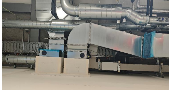
© safetyfocus GmbH – Sealing of ventilation
